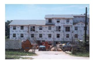
to be postponed. Problems encountered included 1) units not being sufficiently competed for accurate testing, and 2) excessive infiltration beneath baseboard trim above sub-floor; beneath and around kitchen cabinets; and at electrical outlets, bath exhaust fans, window edges, HVAC supply registers, and washer boxes.
